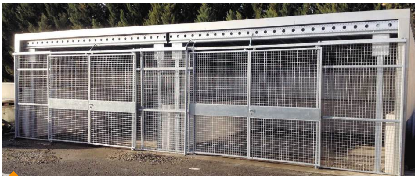
Outdoor shelter using double sliding doors.
