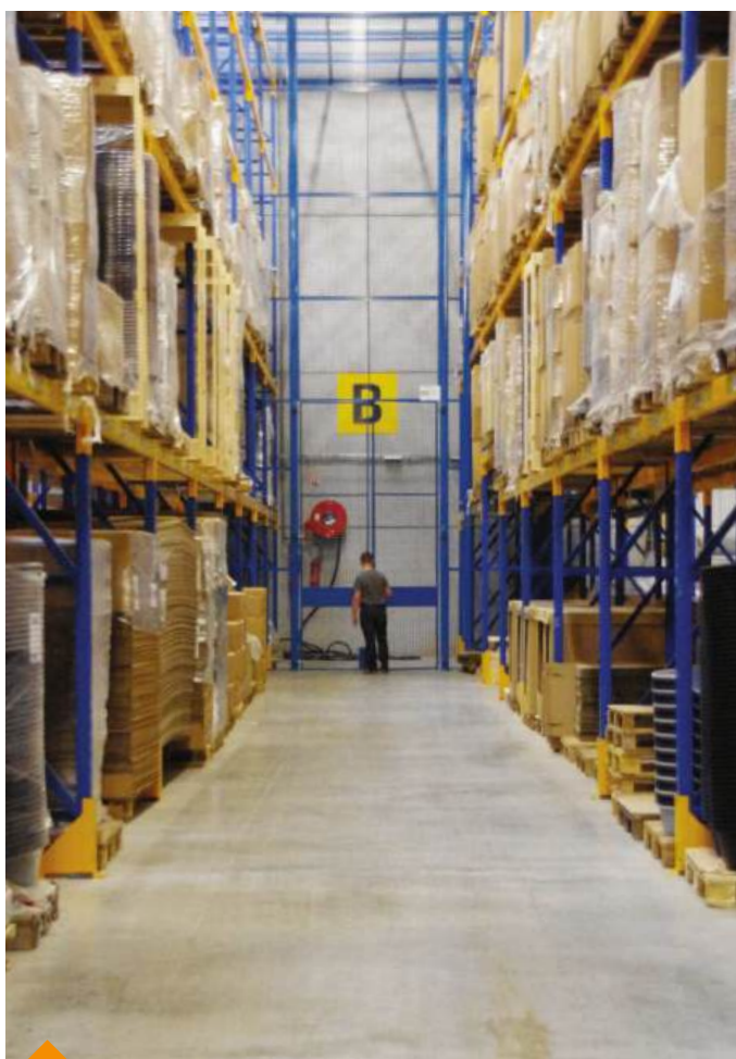
Secured area with double hinged door 4000 mm high and mesh roof.
