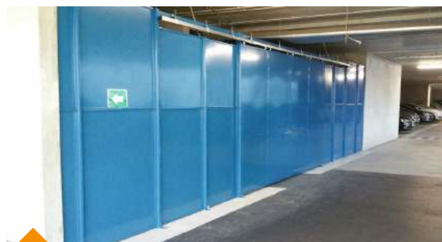
Maintenance area concealed by non-see-through partitions in an underground carpark.
