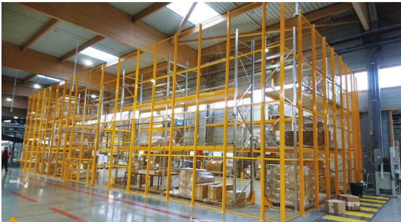
6000 mm high storage area.
