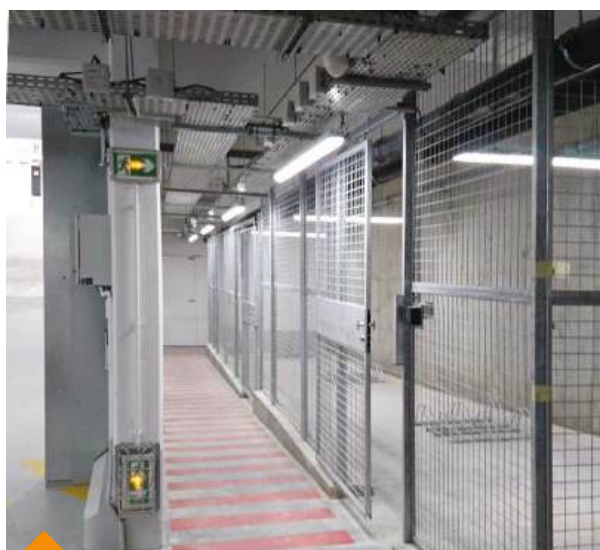
Creation of a storage area in a damp environment and compensation for a sloping floor.
